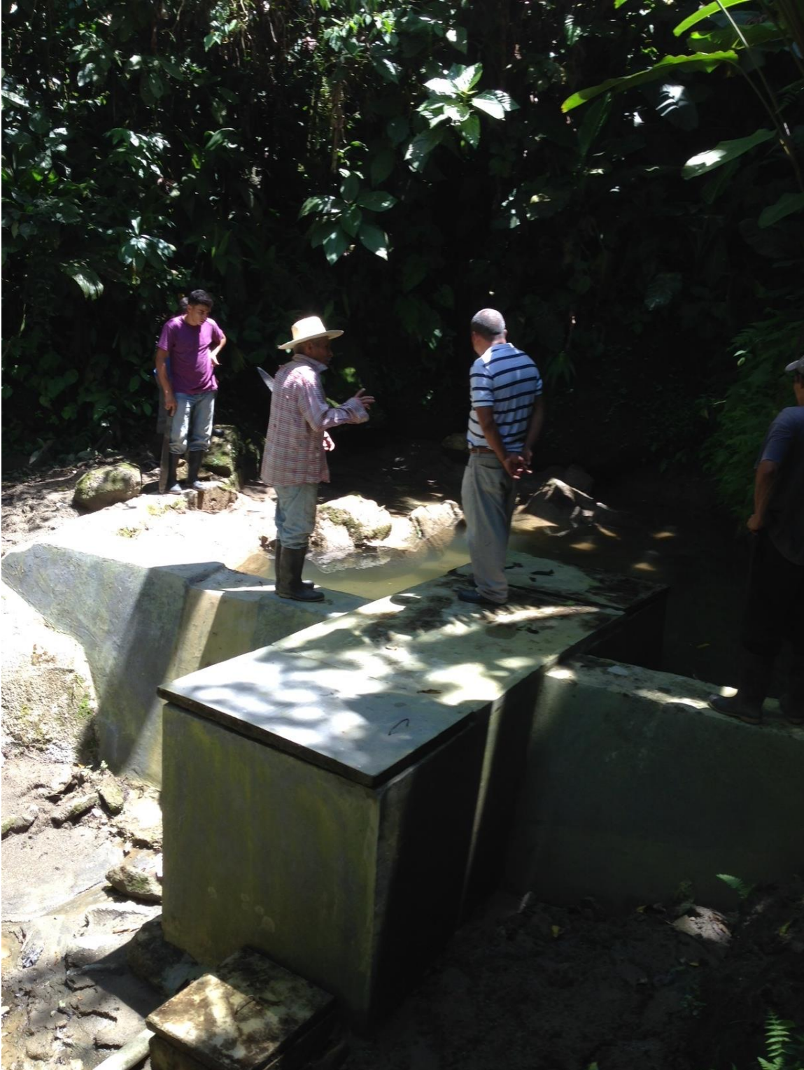
Las Palmas dam. The grouted fissure is between the two men in the foreground, at the waterline.
