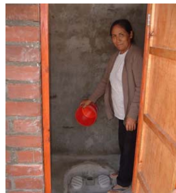
A resident demonstrating the use of the new pour-flush toilets
