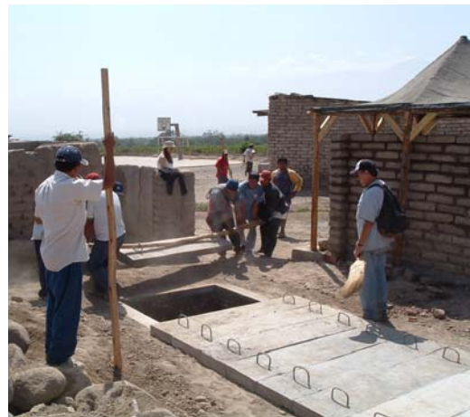
Placing concrete cover sections over the seepage pit
