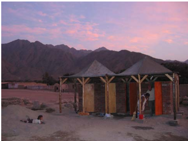
A view of the nearly completed toilet building from the front.
