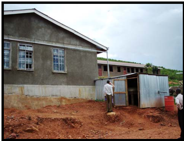
Figure 3 - The rain harvesting system at the secondary school
