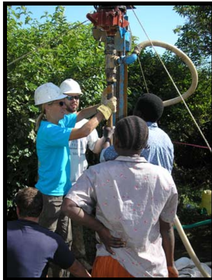
Figure 5 - Drilling with LS-100
