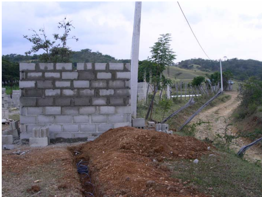
Figure 5-1.2 Main Masonry Storage Tank in Los Cerros
