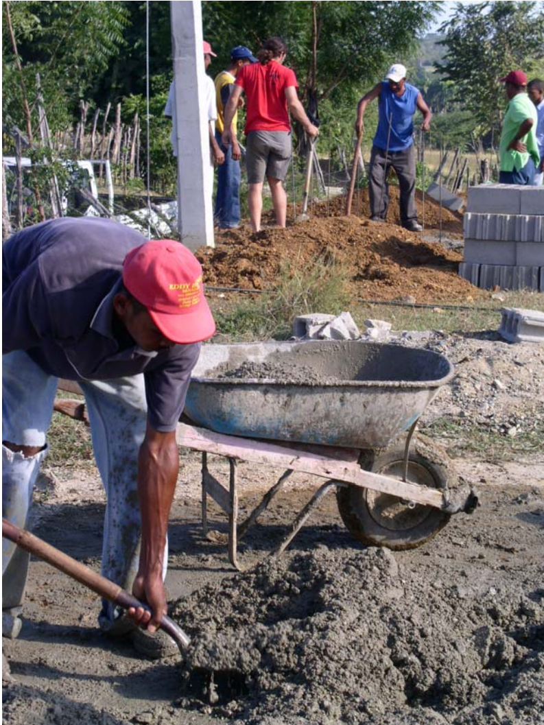
Figure 5-3.1 Community Members Building Storage Tank
