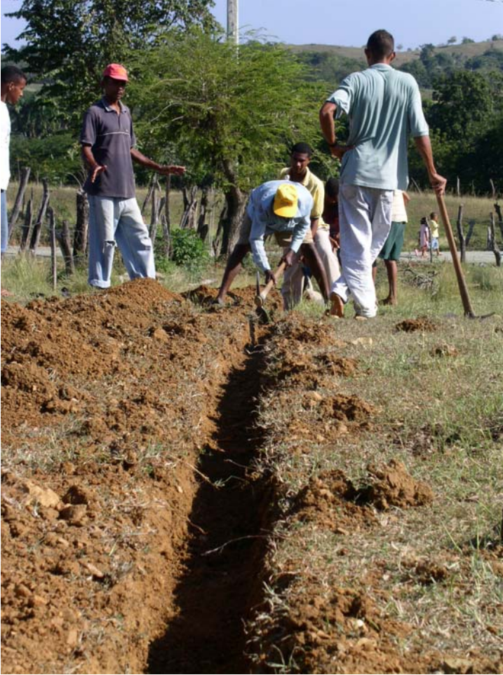
Figure 5-3.2 Men in Community Digging Trench
