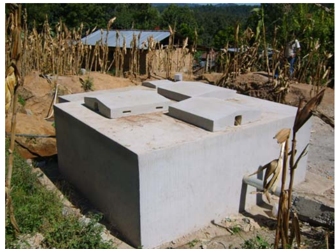
Catchment tank construction(above) and completion.
