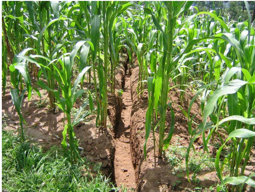
Extensive negotiations for rights of way through many privately owned plots were completed prior to the onset of pipeline placement.
