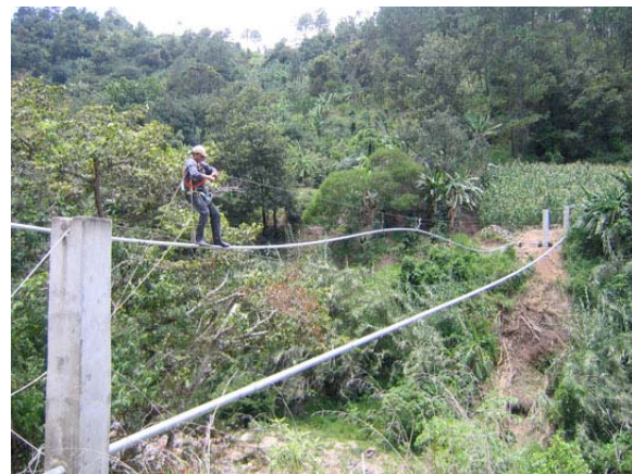
Hanging bridge for water pipe
