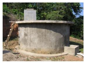
hill above the town. Granular chlorine is added as a water treatment from a hypochlorinator located on top of the main storage tank. The chlorinated water is piped from storage tank to a standpipe at each home through a buried distribution system.
