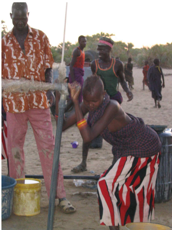
Photo of Water For All manual well drilling method – drilling well in Turkana, Kenya
