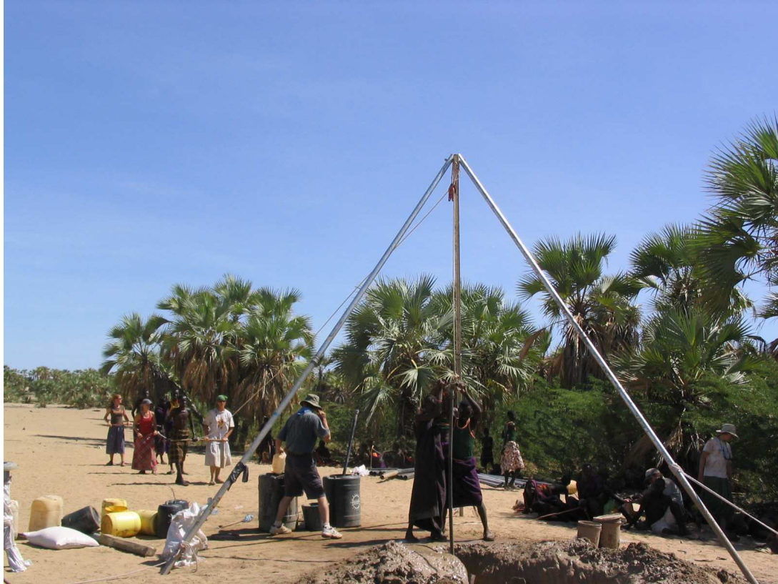
Photo of Water For All manual well drilling method – drilling well in Turkana, Kenya
