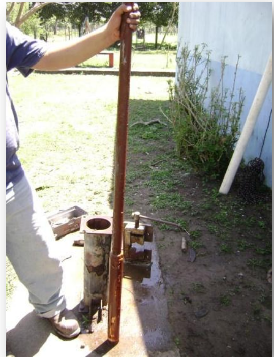
The cylinder pump and riser main are shown as being rusted.
