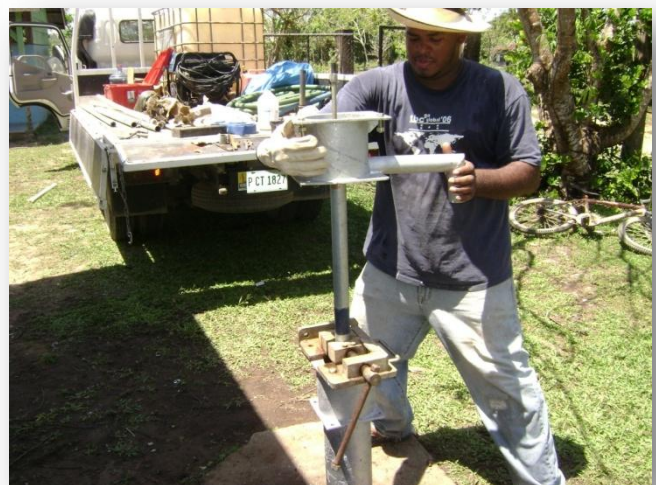
LWI Honduras repair team putting the India Mark II pump together and installing it.
