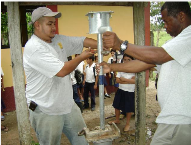
LWI Honduras repair team putting the India Mark II pump together and installing it.
