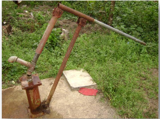
The pump and cylinder rusted
