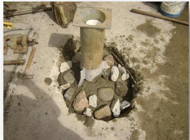
The new India Mark II pump base inserted into the concrete.
