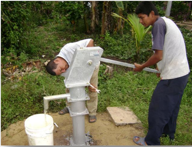
Tightening up the hand pump and testing the handle.
