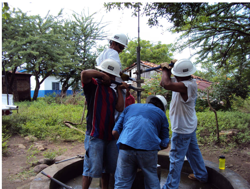
Installing the pump rods.
