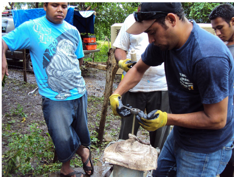
Installing the pump rods.
