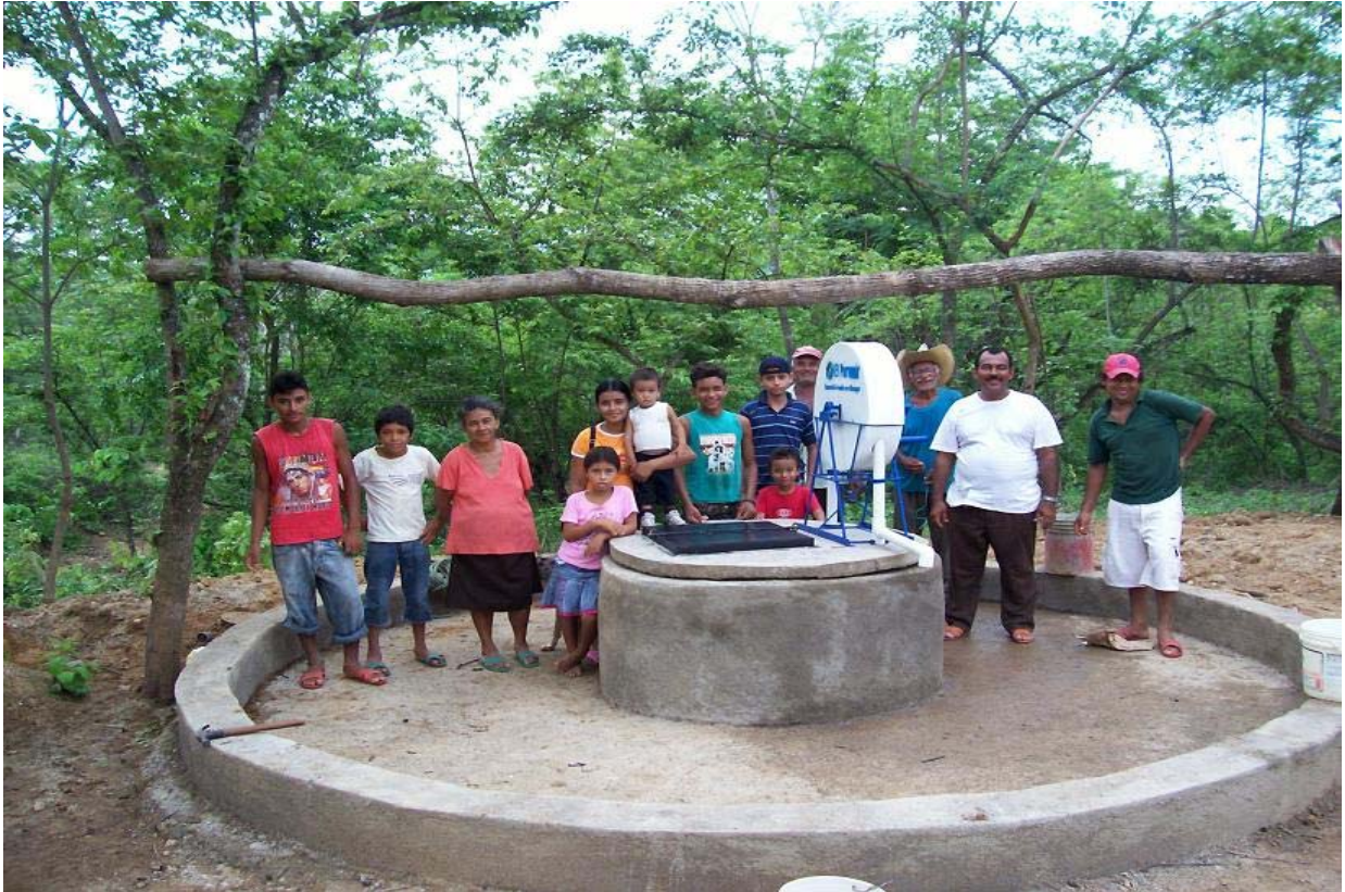
Figure 1: New Hand-Dug Well with Rope-pump and Community Members in Ivan Vilchez Cooperative
