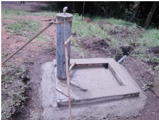
Final construction of a household tapstand, including drainage
