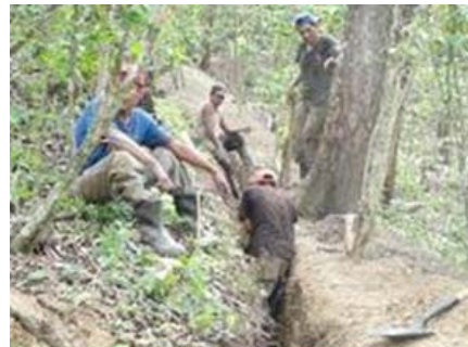
Conduction line trench
