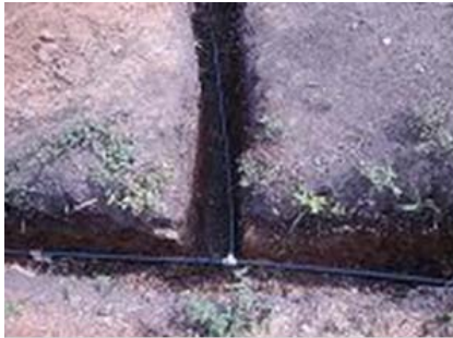
Trench and pipe of the distribution system
