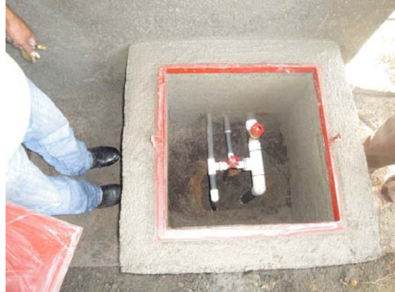
Bypass connection of the storage tank
