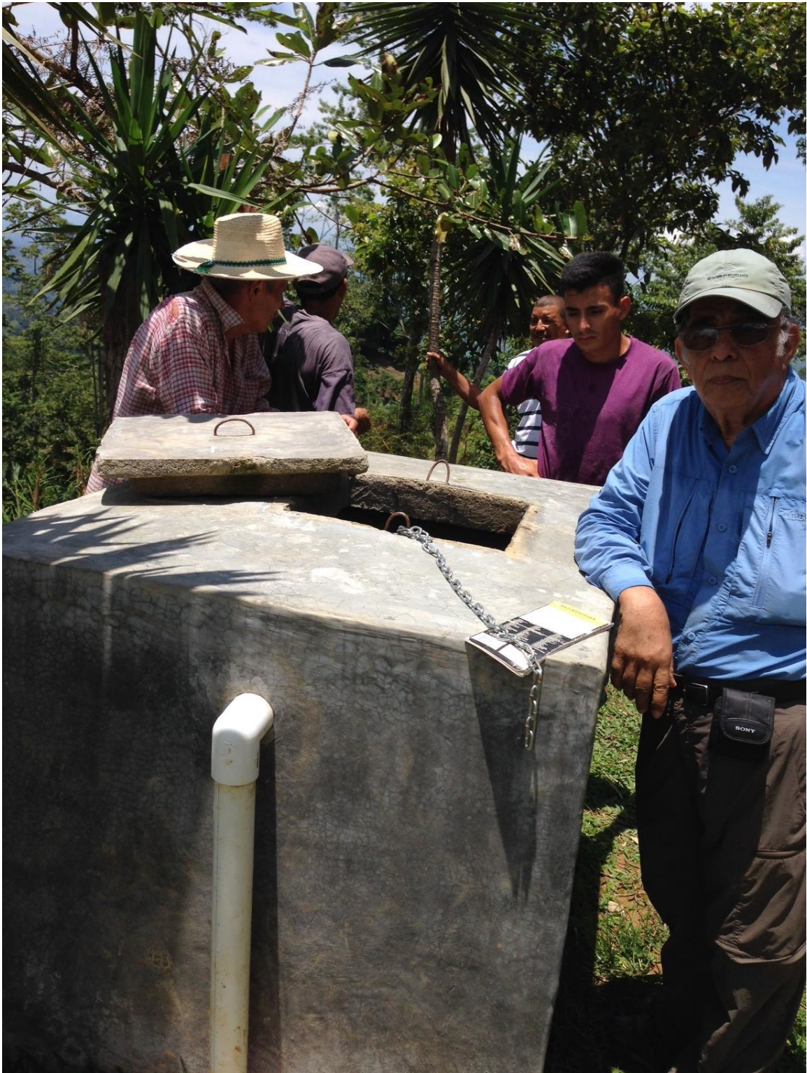
Las Palmas pressure break tank. Rolando López is on the right.
