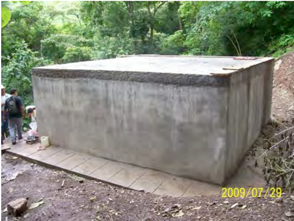
Figure 2: New distribution tank (lower) in Payacuca
