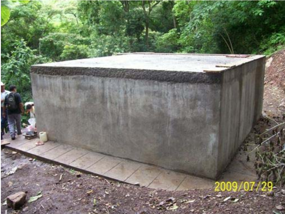
Figure 2: New distribution tank (lower) in Payacuca
